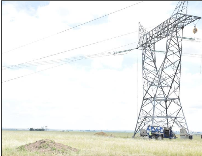
Figure 2: Getting ready for stringing.
